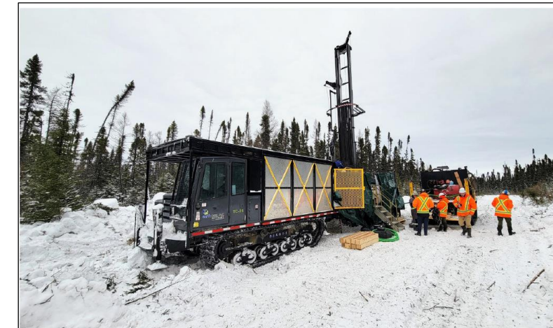
Figure 1: Wallbridge Geologists visiting Earth Drilling's LS600 sonic drill during the February 2023 sonic program.
